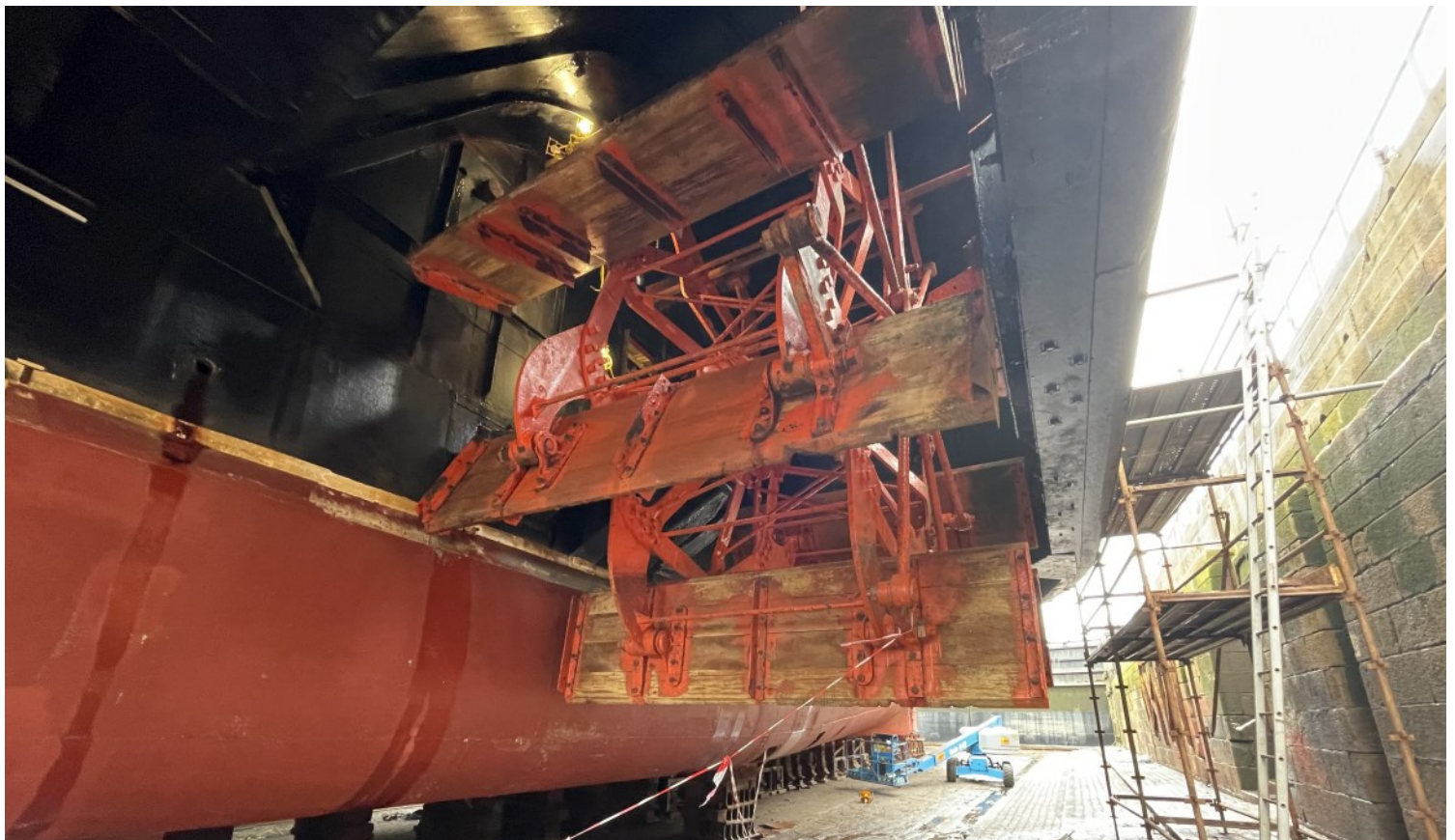
Waverley's port paddle wheel viewed from the dock floor during the 2023 dry docking.
