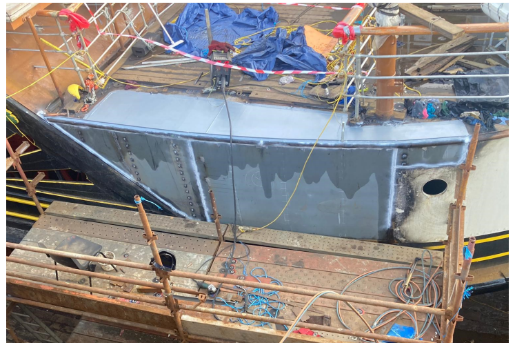
The new shell plating on the port paddlebox.
