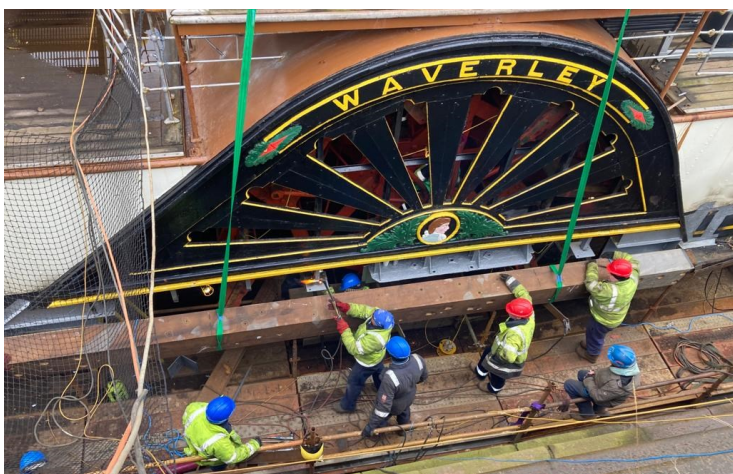
Once steel work was completed the new spring beam was fitted.
